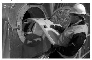
3) ) Insert entire surface of RS in the manhole so that the engaging back plate is caught behind a flanged edge (pic.2). Try to match the flange holes with the oval holes on RS.
